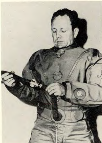
Air entrance assembly, with quick disconnect and sealing hose snapped over entrance port.
