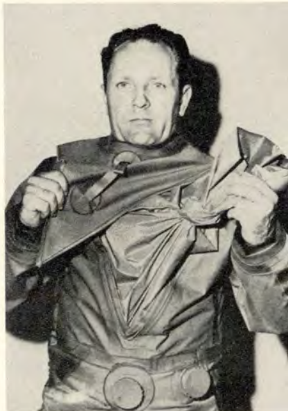
The V-closure, with the zippered flap opened, illustrates how the water barrier is knotted.
